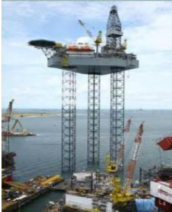
Figure 8: Favelle Favco cranes on Keppel FELS B-Class jack-ups
