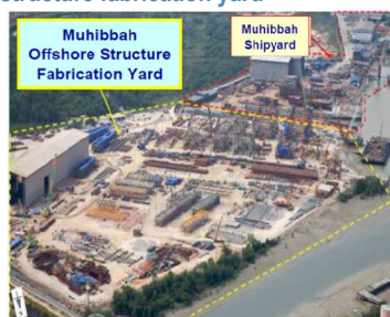
Figure 7: Muhibbah's offshore structure fabrication yard
